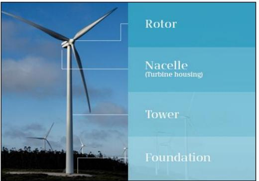
Plate 3-1 Wind Turbine Components.
