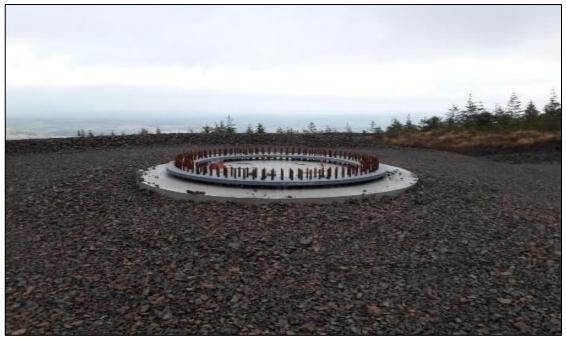
Plate 3-4 Turbine Foundation Back-fill Complete
