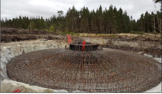
Plate 3-2 Turbine Base 'Anchor Cage'
