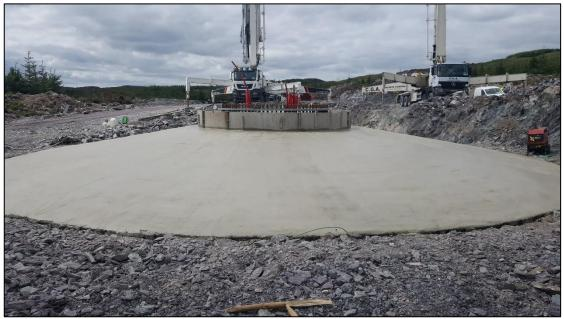
Plate 3-3 Turbine Foundation Poured
