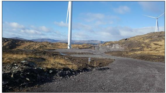
Plate 3-5 Access Road at the entrance to Turbine no. 10 with Turbine no. 9 and hardstand area arrangement in the background
